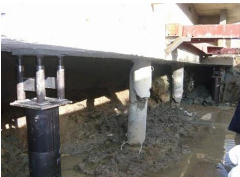
Figure 4: Damage of pile head in Sendai, Miyagi [Masanori Iiba et al., 2012]
