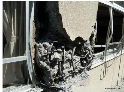
Figure 6: Damage of column buildings in Minami Soma, Fukushima [Kabeyasawa, 2012]
