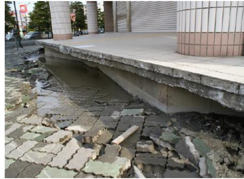
Figure 5: Ground settlement in Urayasu, Chiba [Kohji Tokimatsu et al., 2012]
