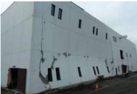
Figure 3: Damage of RC wall in Sendai, Miyagi [Kabeyasawa, T. et al, 2012]
