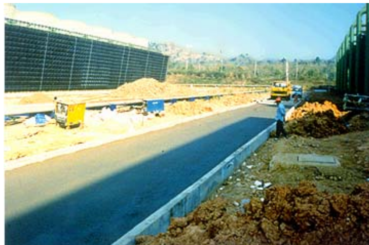
Fig.6 Demonstration construction of Roller-Compacted Concrete Pavement using fly ash at Mae Moh power generating plant
