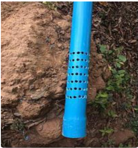
Figure 7: PVC pipe projected borehole
