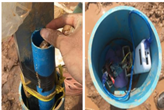
Figure 8: Fill up soil in to borehole
