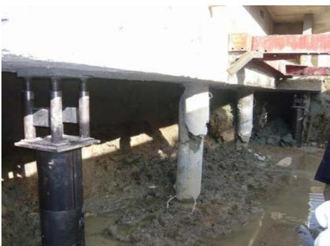
Figure 4: Damage of pile head in Sendai, Miyagi
