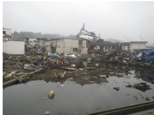
Figure 5 Building damage due to earthquake and tsunami followed by fire in Kesenuma
