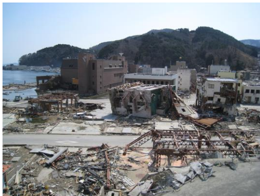
Figure 3 Overall damage from earthquake and subsequent tsunami in Onagawa
