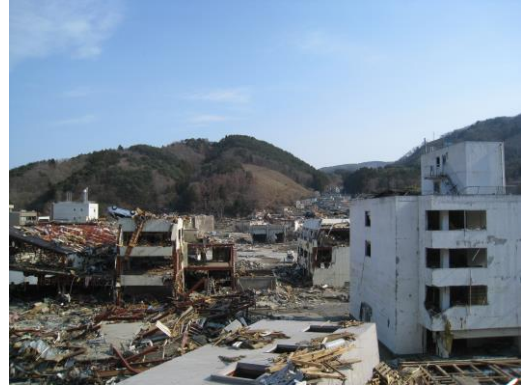
Figure 4 Damage magnifying by the debris impact in Onagawa
