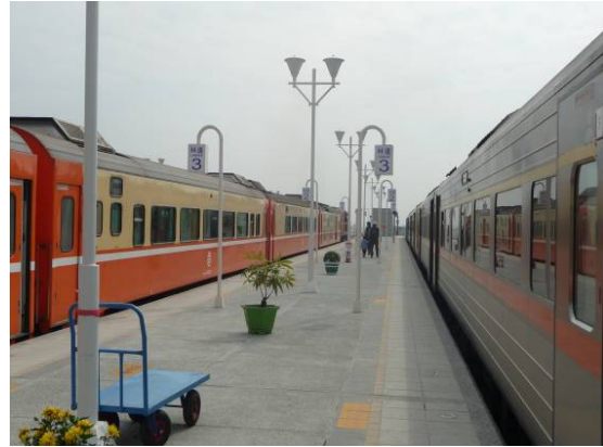
(Fig. 17) New Elevated Platform of Linbian Railway Station.
