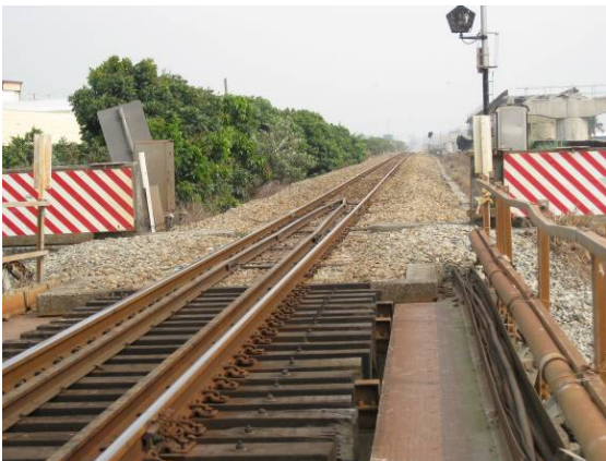
(Fig. 4) Old Water Gate of Linbian River Bridge Dyke Gap
