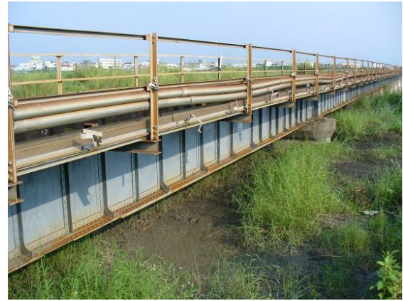
(Fig. 2) Linbian River Bridge before Typhoon Morakot (1)
