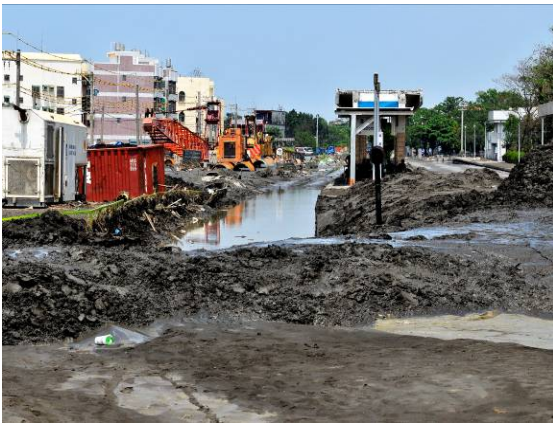
(Fig. 7) The height of deposited soil in Linbian Railway Station was almost as high as the platform.
