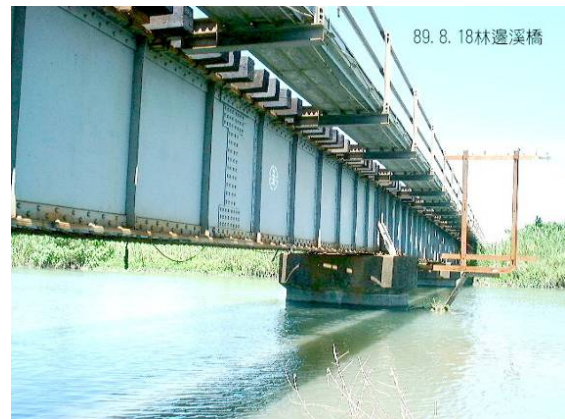
(Fig. 3) Linbian River Bridge before Typhoon Morakot (2)
