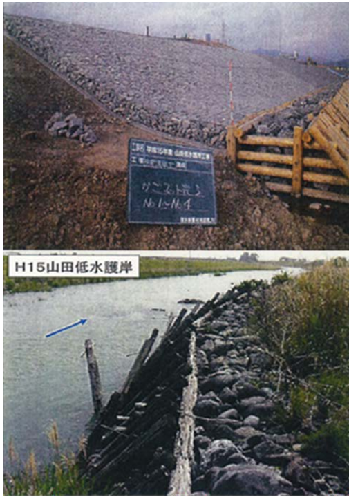
Figure 11 Revetment work constructed in 2003 (top) and current condition (bottom)
