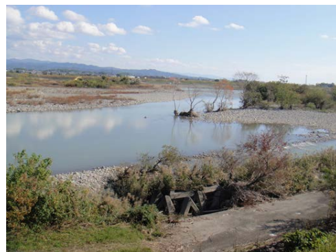
Figure 9 Removal of trees and shrubs in the river channel case
