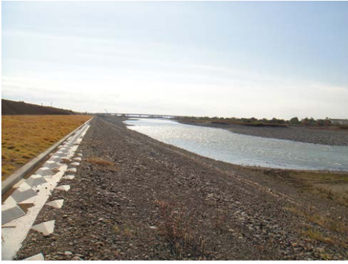
Figure 5 River bank erosion protection and river terrace
