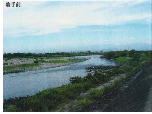
Figure 7 Covering work on river boulders before re-construction
