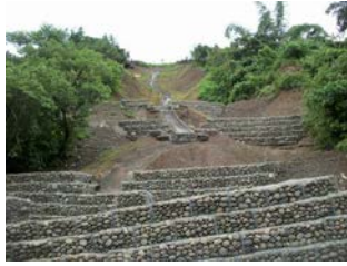
Fig2.5 Landslide remediation project in forest compartment 39 near the Qishan River
