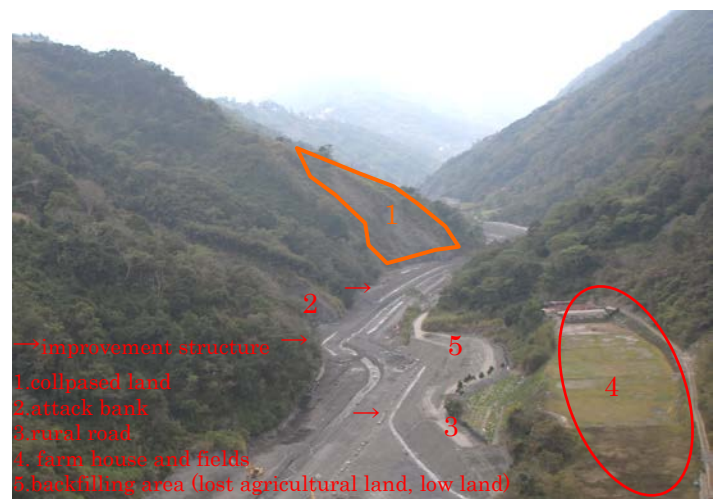
Figure 4-2 The mixing land improvement engineering method improvement structure, showing the objects to be protected
