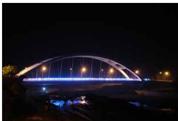
Fig. 17 Night scene of the bridge completion
