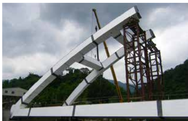
Fig. 15 The Bridge hosting work
