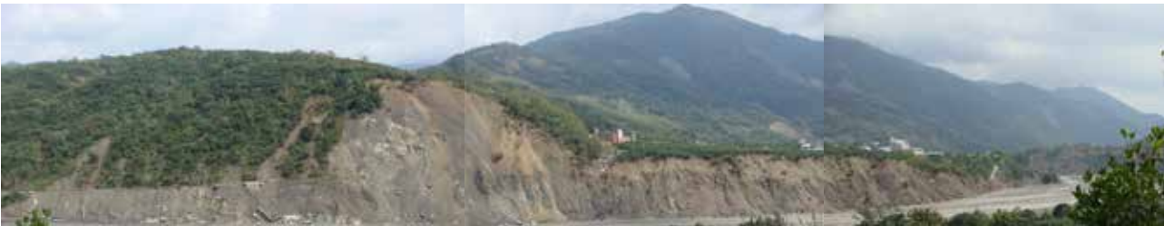
Fig.3 Road damaged after Typhoon Morakot
