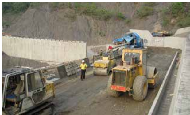
Fig. 13 Road rehabilitation construction
