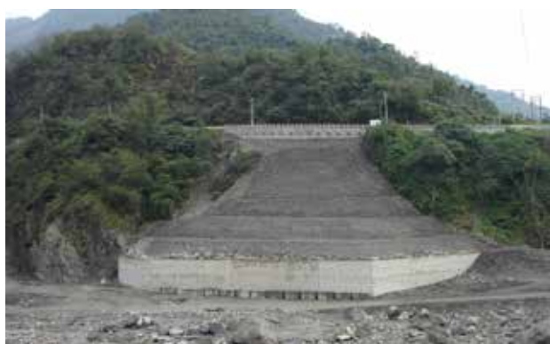
Fig. 14 The River bank protection works
