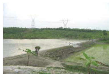
Figure 3. Keruk Situ before collapsed
