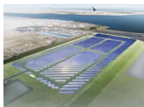
Rendering of the Ukishima Solar Power Plant
