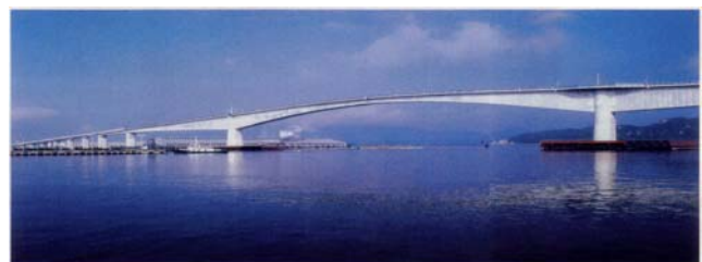
Fig.3 Conventional girder bridge with internal tendon, Eshima bridge, 250m, (Tottori and Shimane prefecture and Kajima)
