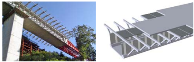
Fig.22 Strutted top slab and corrugated steel webs, incremental launching, Katsurajima bridge, (JH and Sumitomo)
