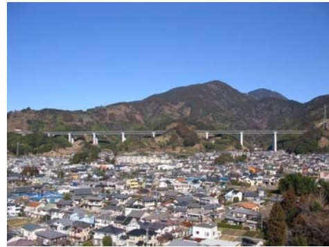
Fig.10 Steel truss webs, Saruta-gawa and Tomoe-gawa bridge, first expressway bridge, (JH and Ohbayashi)
