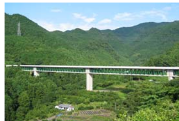
Fig.11 Steel truss webs, Kinokawa bridge, first highway bridge, (MLIT and Kajima)
