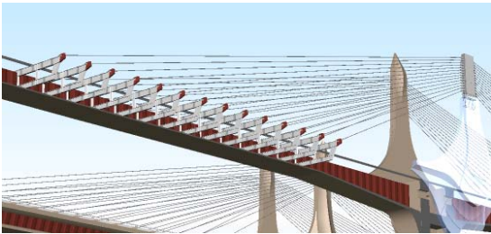
Fig.8 Extradosed bridge with corrugated steel webs, first started construction, Ohmi Ohtori (Ritto) bridge, (JH and PS and Maeda)
