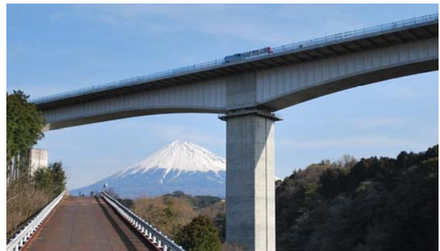
Fig.6 A typical box girder bridge with corrugated steel bridge, Akabuchi-gawa bridge, (Central-NEXCO and Sumitomo)
