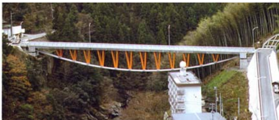
Fig.15 Suspension cable supporting roads above, construction bottom up, Seiun Bridge, (Tokushima prefecture and Sumitomo)
