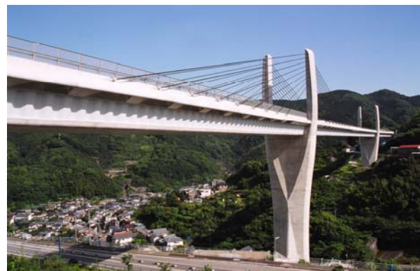
Fig.1 A Typical Innovative Bridge, Himi-Yume Bridge (Nagasaki Prefecture), JH and Mitsui-Sumitomo, Photo by courtesy of Mashiko
