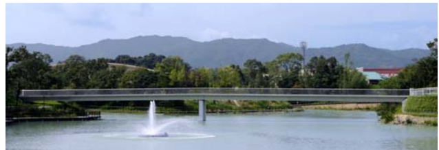
Fig.18 Slender and straight profile of beam by UHPC, Mikane-ike foot bridge, (Ohnojou city, Fukuoka prefecture and Taisei)
