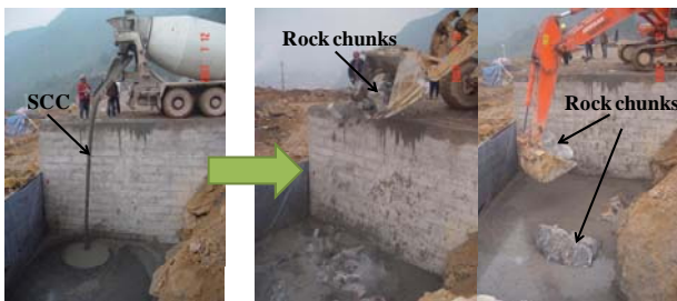
Figure 10 in-situ tests in the Xiangjiaba projects
