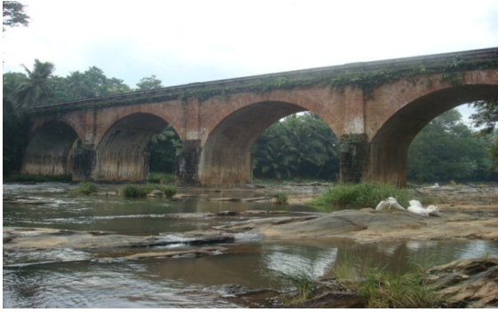
Fig 1 A side view of the A1 90/1 bridge
