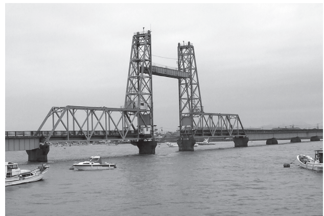
Photo 1.1 Chikugogawa Movable Lift Bridge
