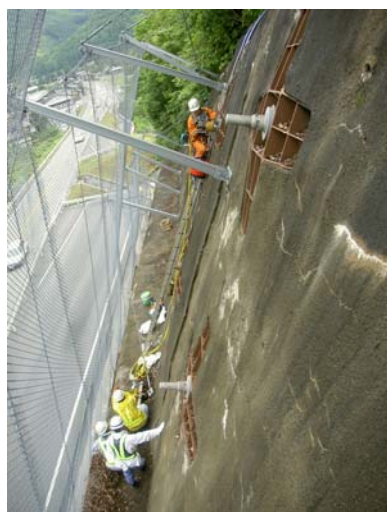
Picture 4. The investigation by new type of the hydraulic jacks
