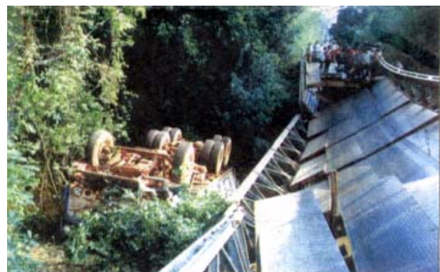
Fig.2 the collapse of a bridge on the road from Siem Reap to Bantey Srey temple on April 10, 2004
