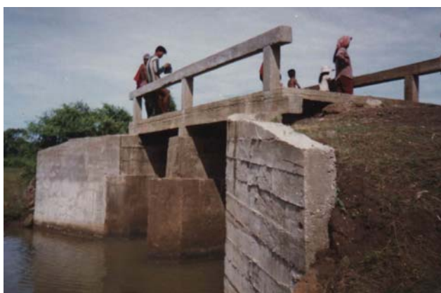
Fig.3 Reinforced concrete bridge
