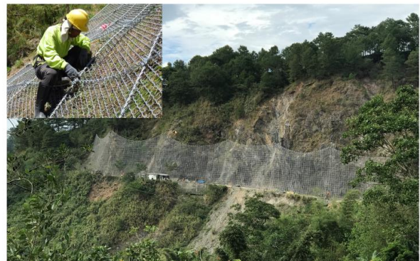
Picture No.1 Pilot Project in Baguio-Tublay
