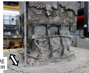
(b) After removing CF-panel and crushed concrete
