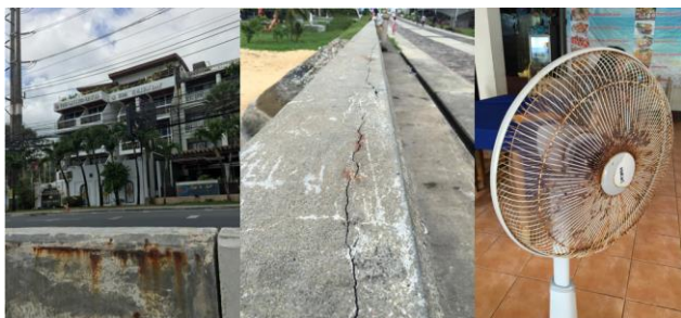
Figure 1.1 Deterioration from airborne chloride
