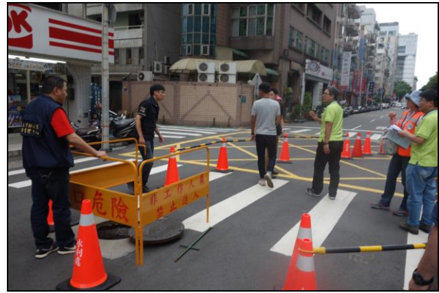
Photo 2.1 Traffic control during storm sewer system inspection.
