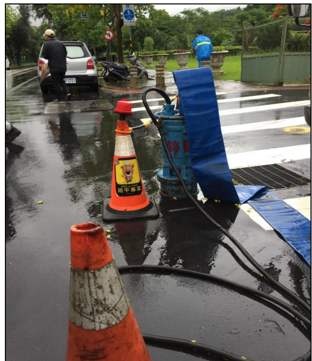
Photo 2.8 The deployment of mobile pump for assisting the capacity of the drainage system.
