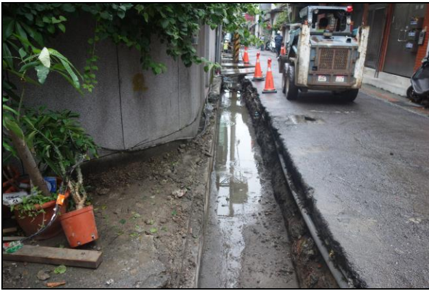
Photo 2.9 Ditch augmentation process to enlarge the capacity of the drainage system.
