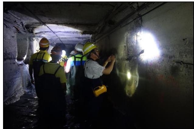
Photo 2.2 Storm sewer system inspection after a flooding instance.
