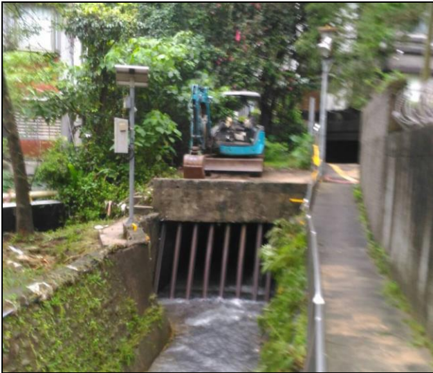
Photo 3.2 The transition channel and the entrance of the sewer system with trash racks at the opening.
