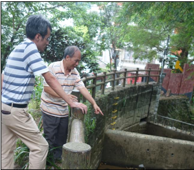
Photo 3.3 The transition channel and the entrance of the sewer system with trash racks at the opening
