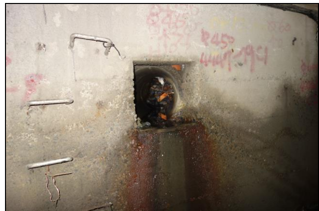
Photo 2.3 A choked pipe which has been marked with painting on the wall during storm sewer system inspection.
