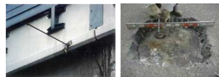
Figure 2: Rupture and protrusion of PC bar (Central NEXCO, 2009)
