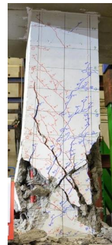
(d) FSF-15S-0.2 Serious damage near the bottom end
