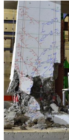
(b) FF-15S-0.2 Concrete spalls severely
