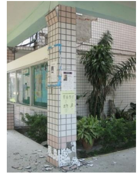
(b) Damage Level III
