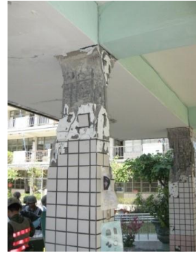
(a) Damage Level IV
