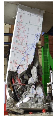
(f) SF-30S-0.2 Serious damage
