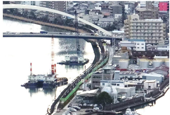
Figure13 Reinforcing of river mouth levees
