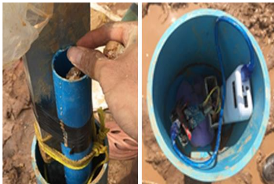
Figure 8: Fill up soil in to borehole
