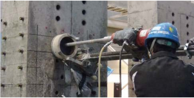
Figure-6 Actual situation (core drilling)
