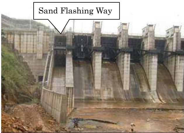
Fig.-15 Sand-Flushing-Way
