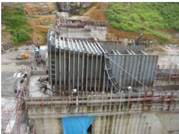
Fig.-17 SCC Placing underneath Sand-Flushing-Way
