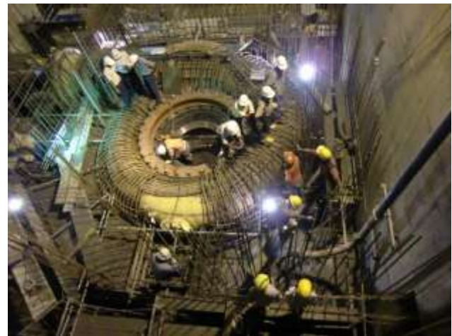
Fig.-18 Spiral Casing in Powerhouse
