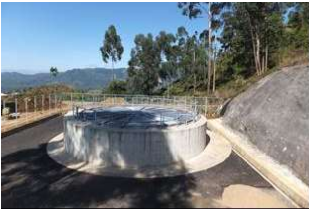
Fig.-3 Upstream Surge Tank
