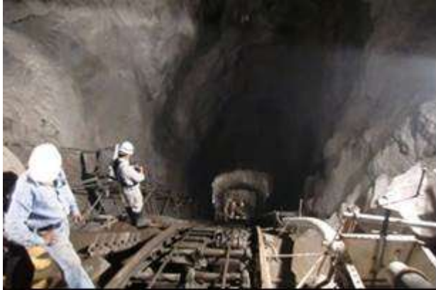
Fig.-4 Inclined Penstock Tunnel
