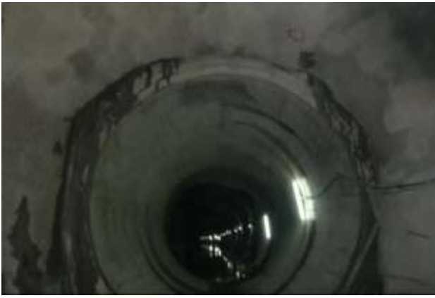
Fig.-2 Headrace Tunnel
