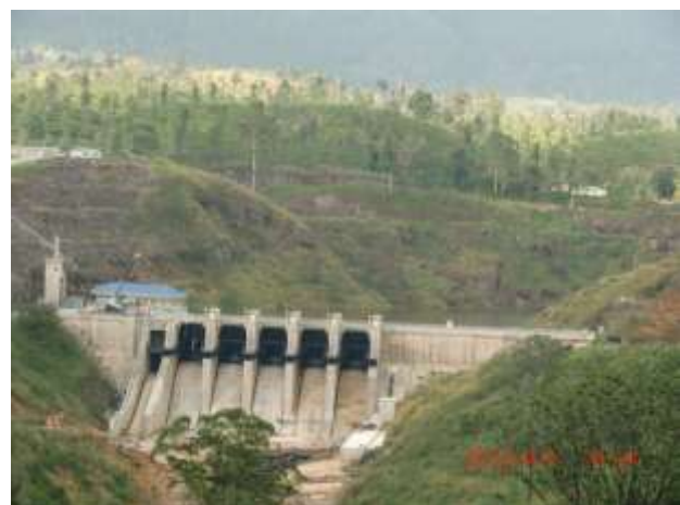
Fig.-1 Intake Dam
