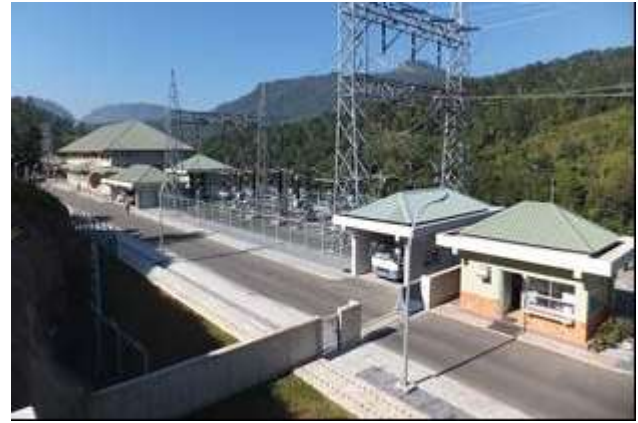
Fig.-6 Outdoor Switchyard and other Facilities
