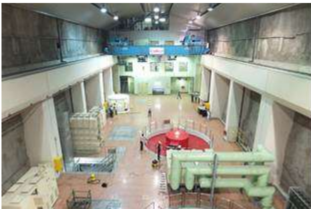
Fig.-5 Underground Powerhouse
