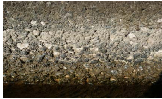
Fig.1 Concrete canal generated exposure of coarse aggregate
