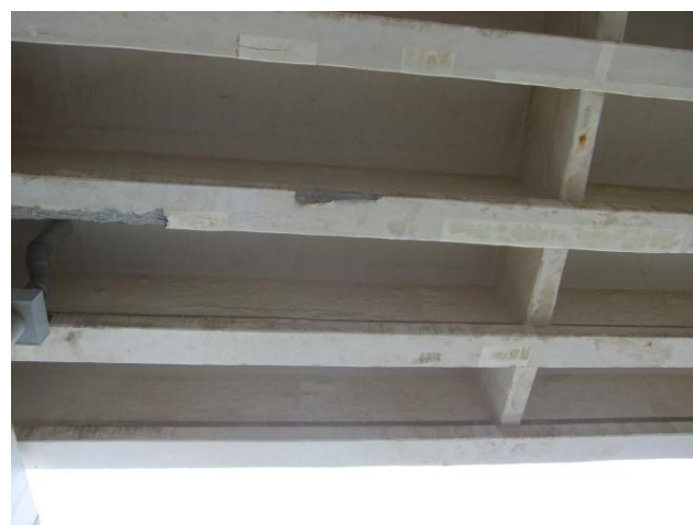
(a) patching and painting (7th span)
