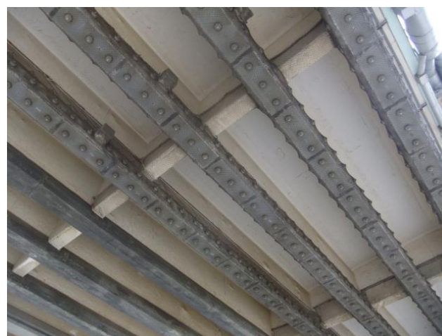
(b) cathodic protection (8th span)
