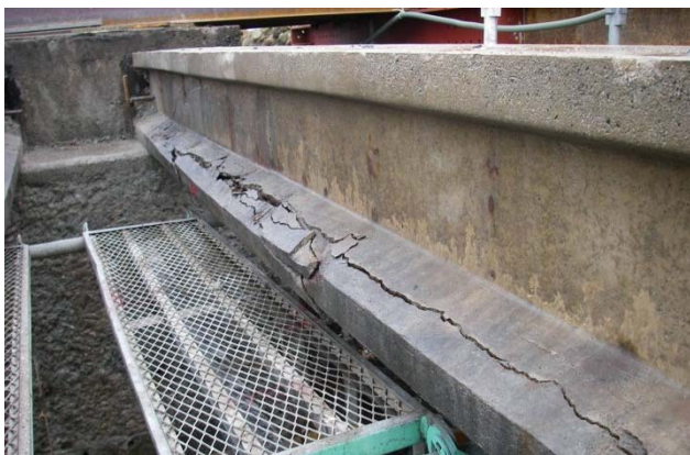
Figure1 an example of deteriorated PC bridge beam affected by salt attack in Niigata pref., Japan (constructed in 1975)
