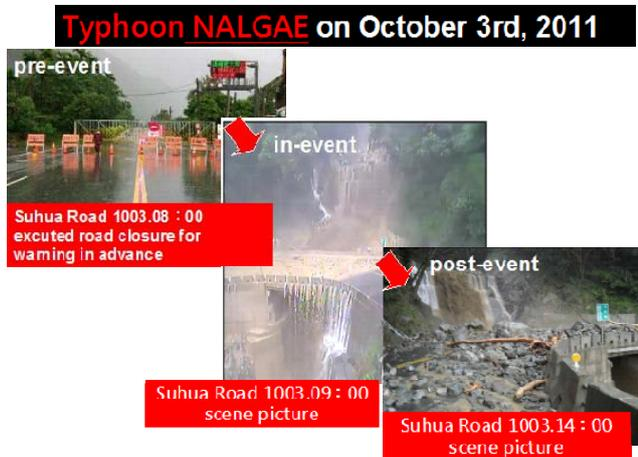
Figure 6 SuHwa highway damages caused by Typhoon Nalgae in 2011.
