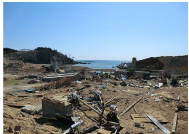
Fig.5 Washed away of concrete bridge
