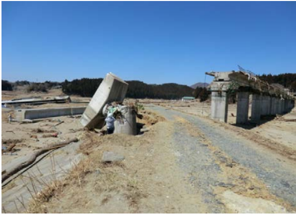
Fig.6 Broken pier at the top
