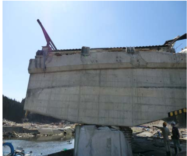
Fig.9 Broken anti-fallen device
