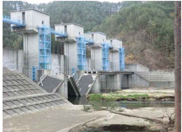
Fig.14 Broken decks next to water gate
