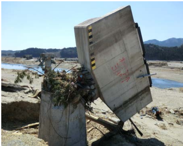
Fig.7 Close-up view of broken pier
