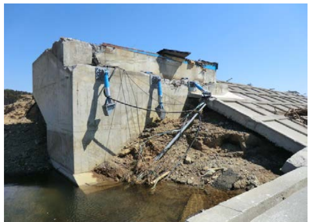
Fig.11 Broken anti-fallen device
