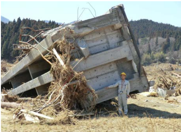
Fig.8 Fallen prestressed concrete girder
