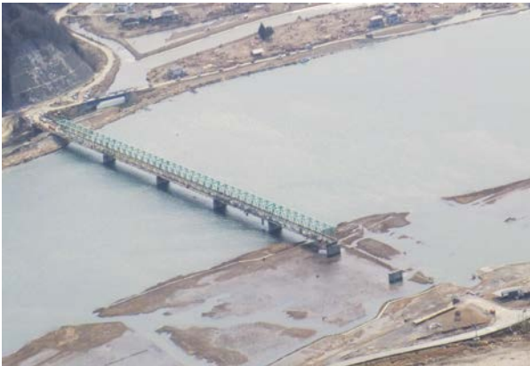
Fig.12 Truss bridge washed away
