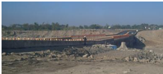
Photo 2.2 Completed temporary access road
