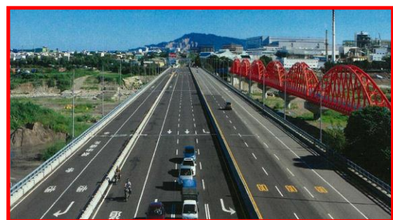
Photo 4.3 Completed Houfeng bridge
