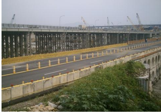
Photo 3.1 Completed temporary access bridge
