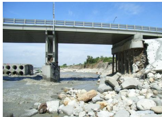
Photo 5.2 Temporary steel bridge with H-section steel pile
