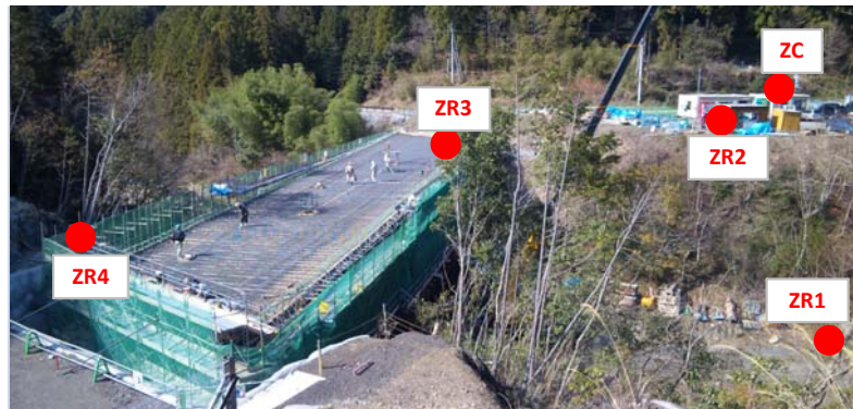
Figure 6 ZigBee Coordinator and Reuters on construction site
