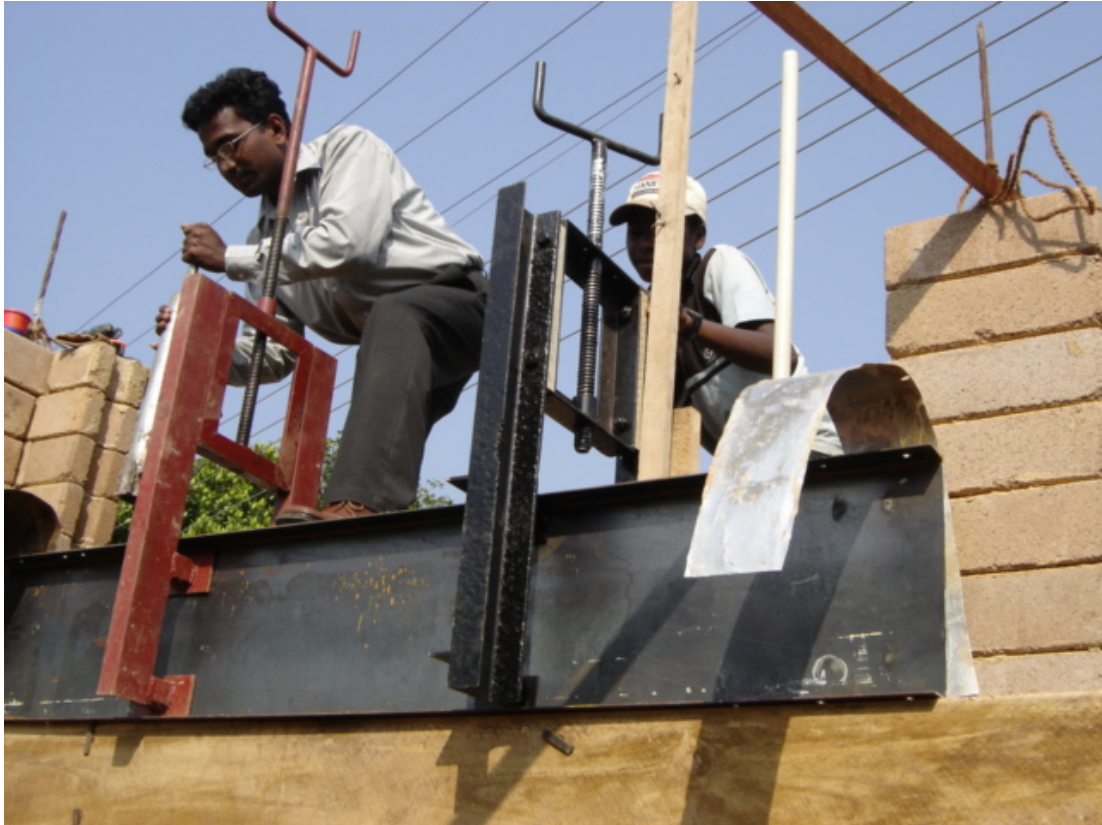
Figure 4: Rammed earth construction
