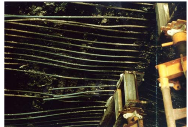
Figure 4.1 Serious damage of concrete slab by fire
