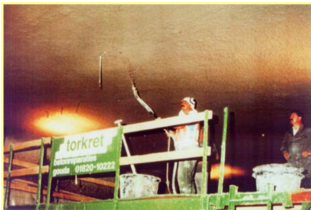
Figure 5.2 Mitigation measures by sprayed fire protection 6)
