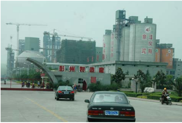
Fig. 18 The concrete pre-mix factory was intact
