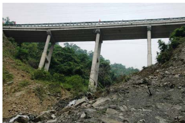
Fig. 30 The damaged bridge in Highway 213
