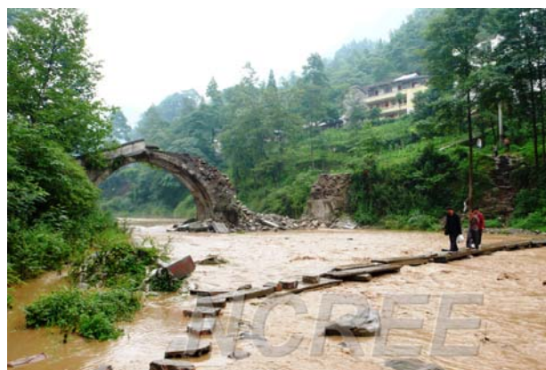
Fig. 29 The destroyed arch bridge in Bailu
