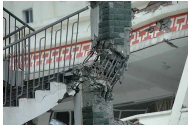
Fig. 10 The close-up of a damaged RC column
