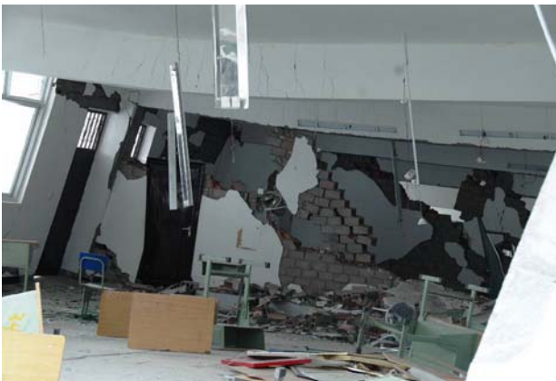
Fig. 8 The damaged classroom
