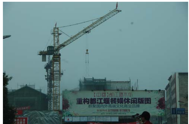
Fig. 22 The crane tower is still in operation
