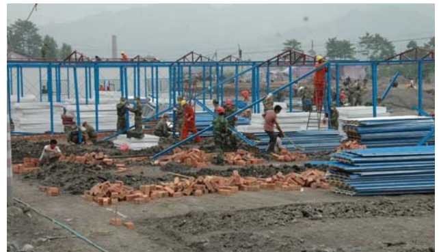
Fig. 42 The temporary houses under construction near Pongzhou.
