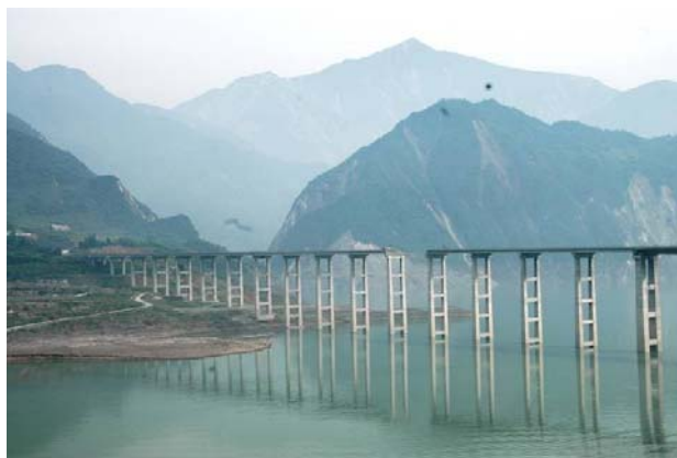
Fig. 28 The falling span of Miaotzuping bridge
