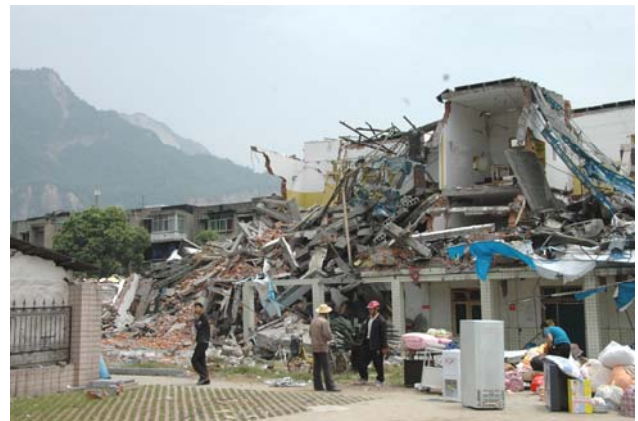
Fig. 11 The collapsed dormitory of a hospital
