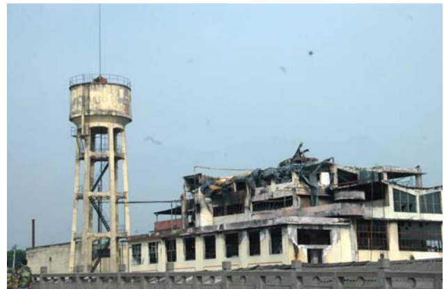
Fig. 21 Another undamaged water tower
