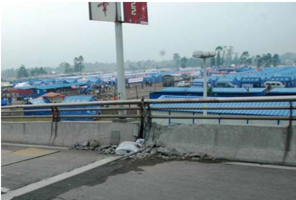
Fig. 32 The damaged expansion joint
