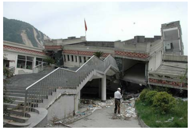
Fig. 9 The collapsed RC school building
