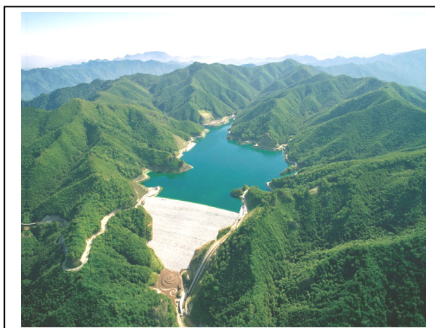
Fig.4.13 Bird's-eye View of Upper Dam
