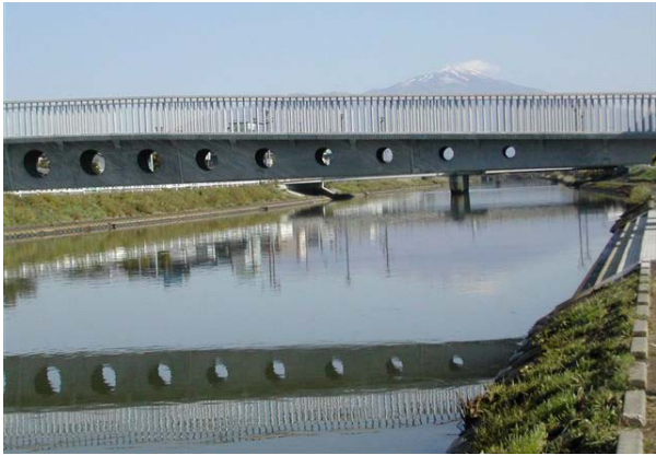
Fig. 8 Sakata Mirai Bridge [10]
