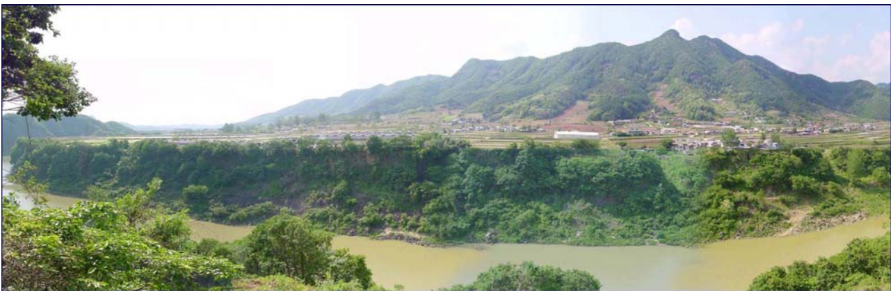
Figure 6 Dam Site for Hantan-gang Dam Grand Design Project (The Republic of Korea)
