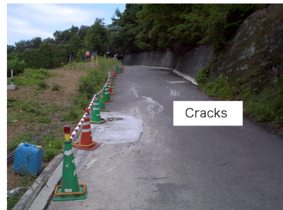
(a) Cracks on the road
