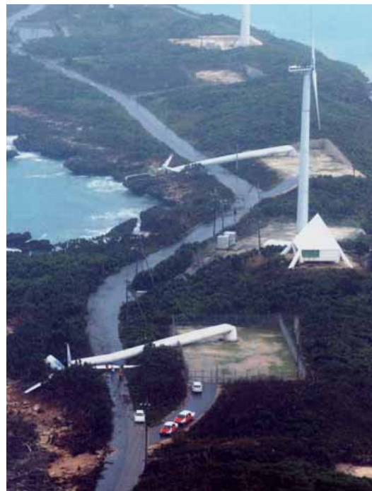
Figure7 damaged wind turbines at Karimata plant (Ishihara et al., 2005a)
